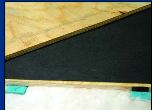
3) Build-up isolated subfloor
