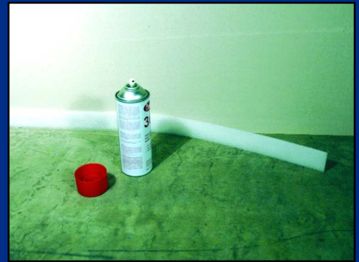
1) Place Perimeter Board (Model SRP)
